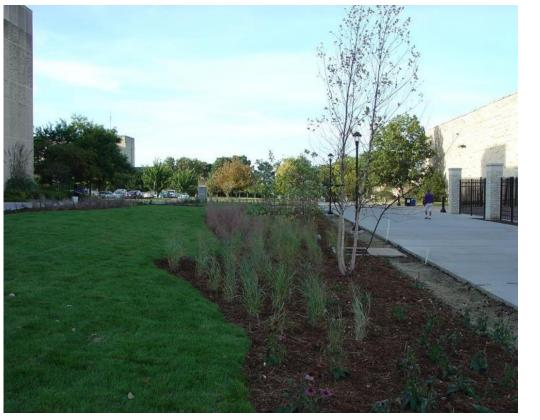
Bio-retention areas along 17<sup>th</sup> Street seek to reduce the impacts of impervious paving and thus slow and infiltrate stormwater runoff.
