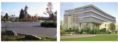
Green (living) roofs, bio-swales & rain garden; Three existing stormwater structures were repurposed as cisterns to capture, store and recirculate rainwater for irrigation. Pervious site pavement allows stormwater to seep into the ground, reducing runoff; Drought-tolerant native & naturalized plant species minimize need for irrigation while creating habitat within the city.
