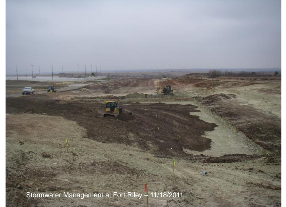
Large bio-retention areas were constructed in 2011 and 2012 as an attempt to mitigate the large areas of impervious paving at Fort Riley, KS.
